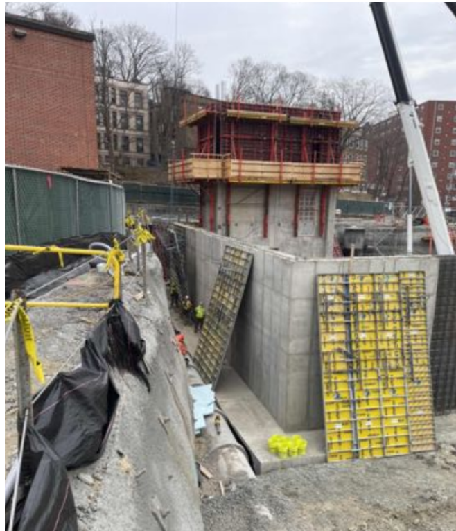
Forming and placing walls along the CY line adjacent to the existing school. (Photo Below)
